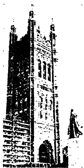
The Victoria Tower, while renovation was still being carried out on the Palace of Westminster. The statue is of King George V.
